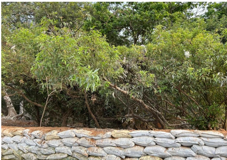
Figure 20: Sandbags alongside the island to prevent flooding. Image Source: Author
